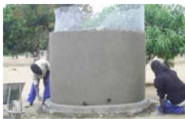
Figure 5: Ferro-cement tanks built on the spot in a remote area in southern Mozambique in 2011
