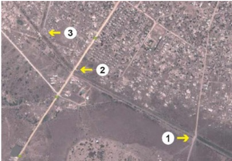
Figure 3: Southern drainage channel (1: location of bridge obstructing the channel; 2: regional highway bridge, which is not an obstruction; 3: T-joint in the drainage channel).
