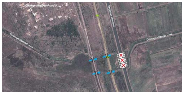
Figure 21: Detail of crossing “2” where the pipes under the irrigation channel are collapsed
