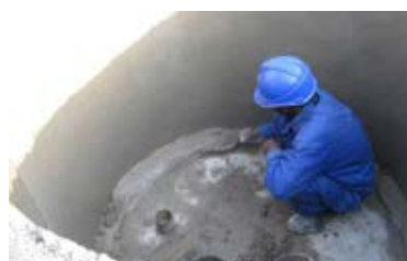
Figure 5: Ferro-cement tanks built on the spot in a remote area in southern Mozambique in 2011
