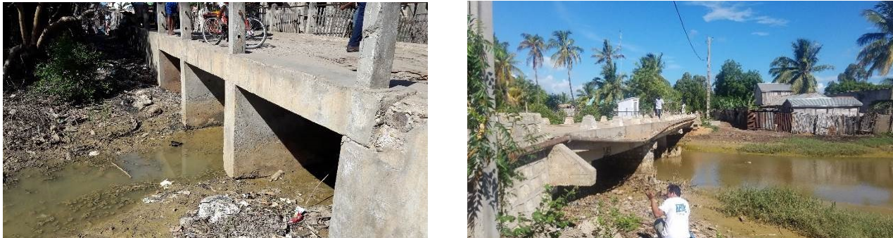
Figure 9: Bridges crossing the Hellot Channel
